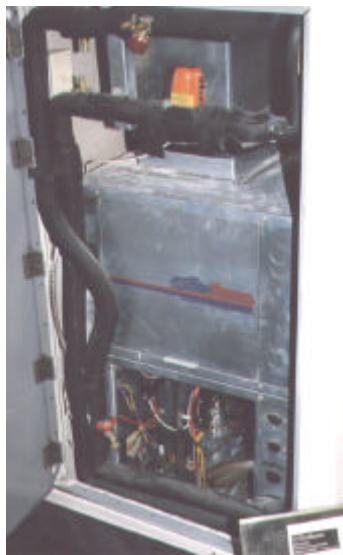
Figure 4. Typical Single Room Heat Pump Unit
